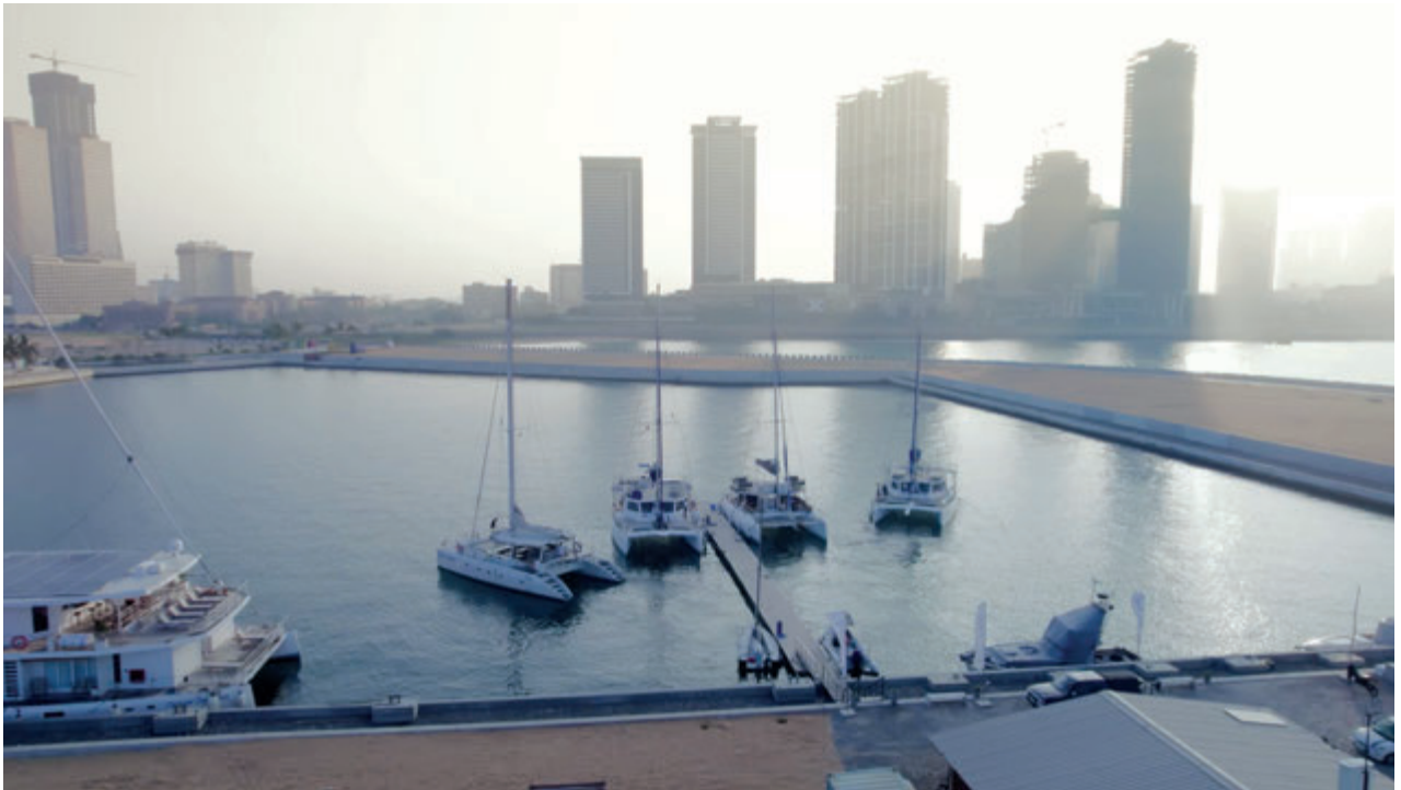
Marinas at Colombo Port City.
