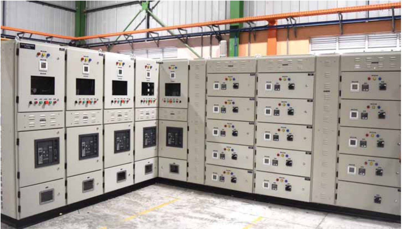
Supply of 4000A Synchronizer Panel for UI Technical, Hakuruhura Project, Maldives
