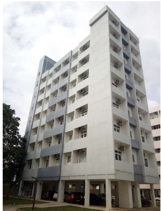
6.11 – Office Single Quarters (Major & Above) - 09 Storey Building
