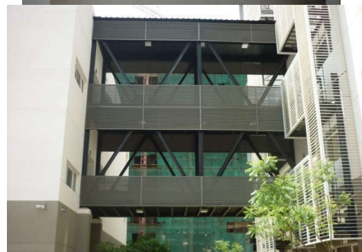
Two Level Steel Bridge between Buildings 3.1 A and 3.1 B
