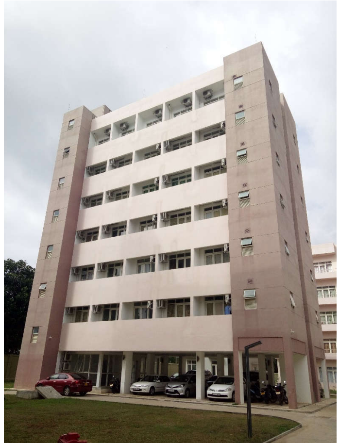
6.9 – Office Single Quarters (Major & Below) - 07 Storey Building
