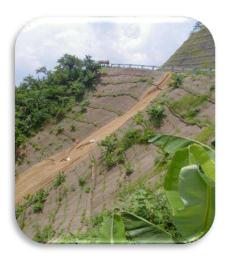
This product, which is 100% Coir & natural rubber latex, is environmentally friendly and totally biodegradable over a period of time. It is ideal for bio technical, and soil bio engineering applications. It is designed to be used as a top soil cover to prevent erosion of soil and enhance the biological aspects of engineering.
