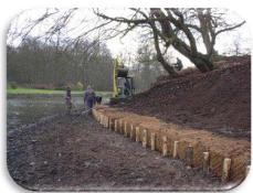
Geo logs of 40 cm x 40 cm rectangular dimension with machine or hand woven nets
