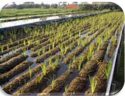
Geo-rolls with woven net, inner lined with rubberized coir pad circular and rectangular sections. stuffed with a mixture of Coir pith and Coir fiber. Dimensions of the bio rolls can be made to specifications
