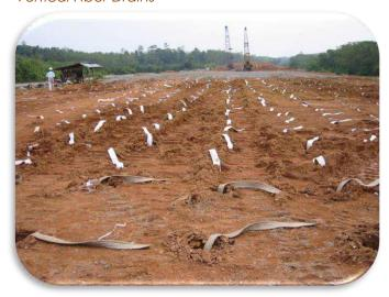
Natural fabricated Vertical Fiber Drains (VFD's) produced from biodegradable materials such as jute and coir have some distinct advantages over conventional polymeric prefabricated vertical drains (CPVDs). For instance, VFD's are not only able to discharge excess pore pressure effectively, but are also beneficial to the environment thanks to their biodegradability.
